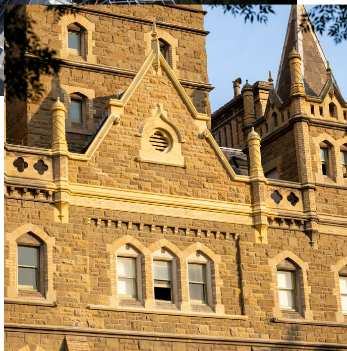
Images: Stone restoration works on the Main Building.
